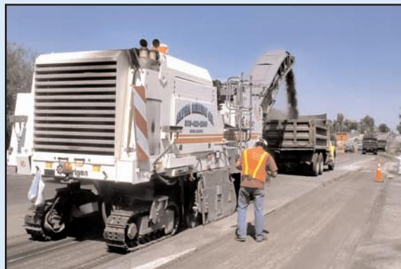
The **Wirtgen W 2000** from Wirtgen America is a high-performance, large-volume, compact milling machine with broad cutting width for removing deteriorated asphalt pavement or complete roadway structures down to 13 inches in a single pass. The W 2000 boasts a 565 hp engine and features front loading of RAP for ease of operations. It has a base cutting width of 79 or 87 inches, can operate at speeds up to 180 fpm, and has an operating weight of approximately 64,000 pounds.
