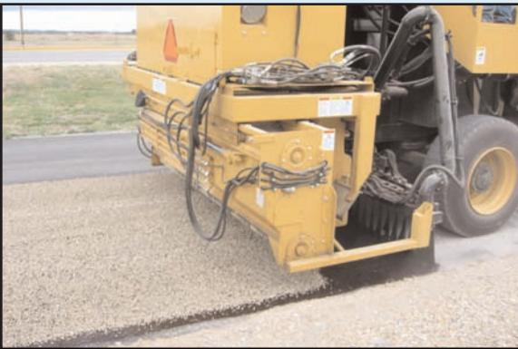
**RoadArmor High Performance Chip Seal** is a single pass surface treatment developed for cost-effective pavement preservation with low user delays. It is designed for high traffic roads in good condition but with minor surface distresses. A new ultra-fast setting polymer modified emulsion is used with a single-sized aggregate in a continuous synchronized application. RoadArmor surfacing means quick traffic return, reliable performance, and low risk of vehicle damage.
