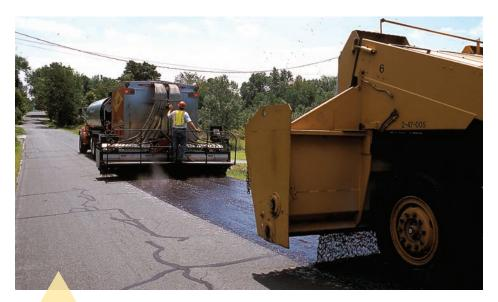
Crack sealing prior to applying a surface treatment reduces moisture damage.
